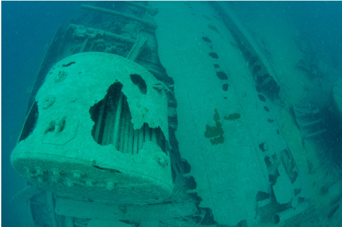
Figure 9: Boiler with fire tubes inside visible (the engine mountings can be seen standing up behind, and to the right of the picture the second boiler is just in view)
